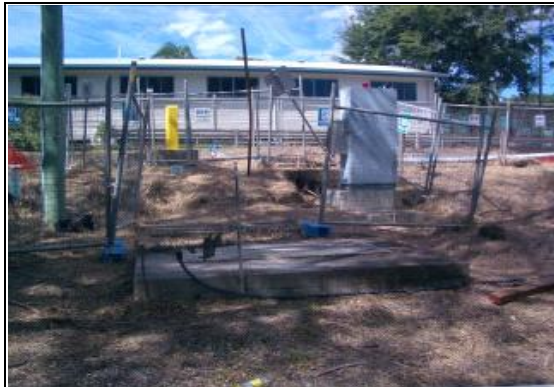
Existing Pump Station
