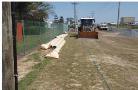
Pipe laying (North of Commercial Ave)
