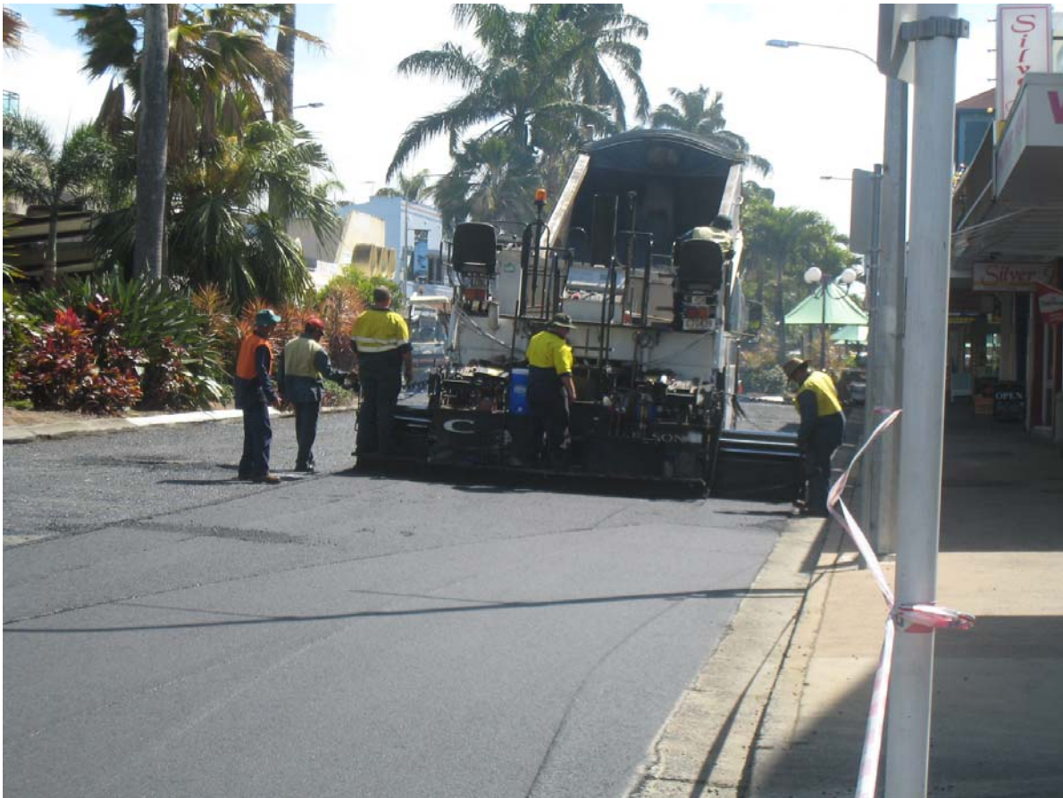
Wood Street Final Surfacing
