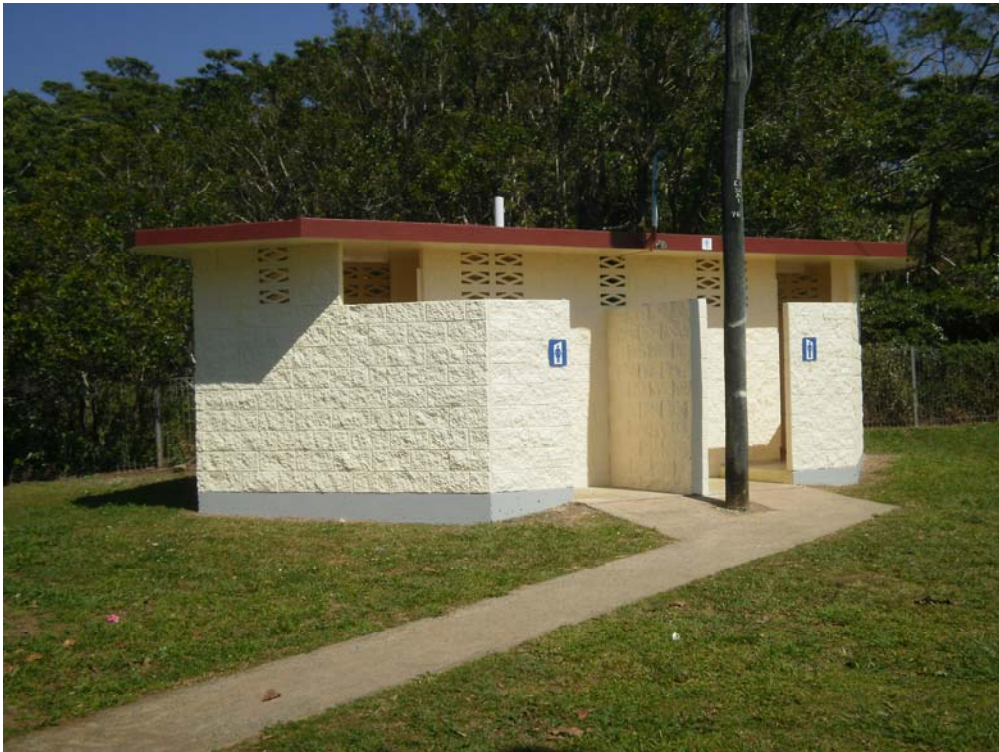
Eungella Amenities Refurbishment
