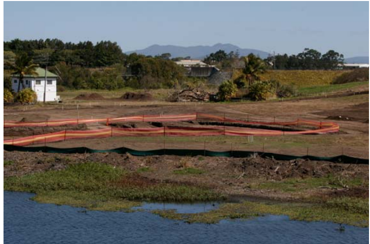
Outdoor Performance and Events Centre - earthworks
