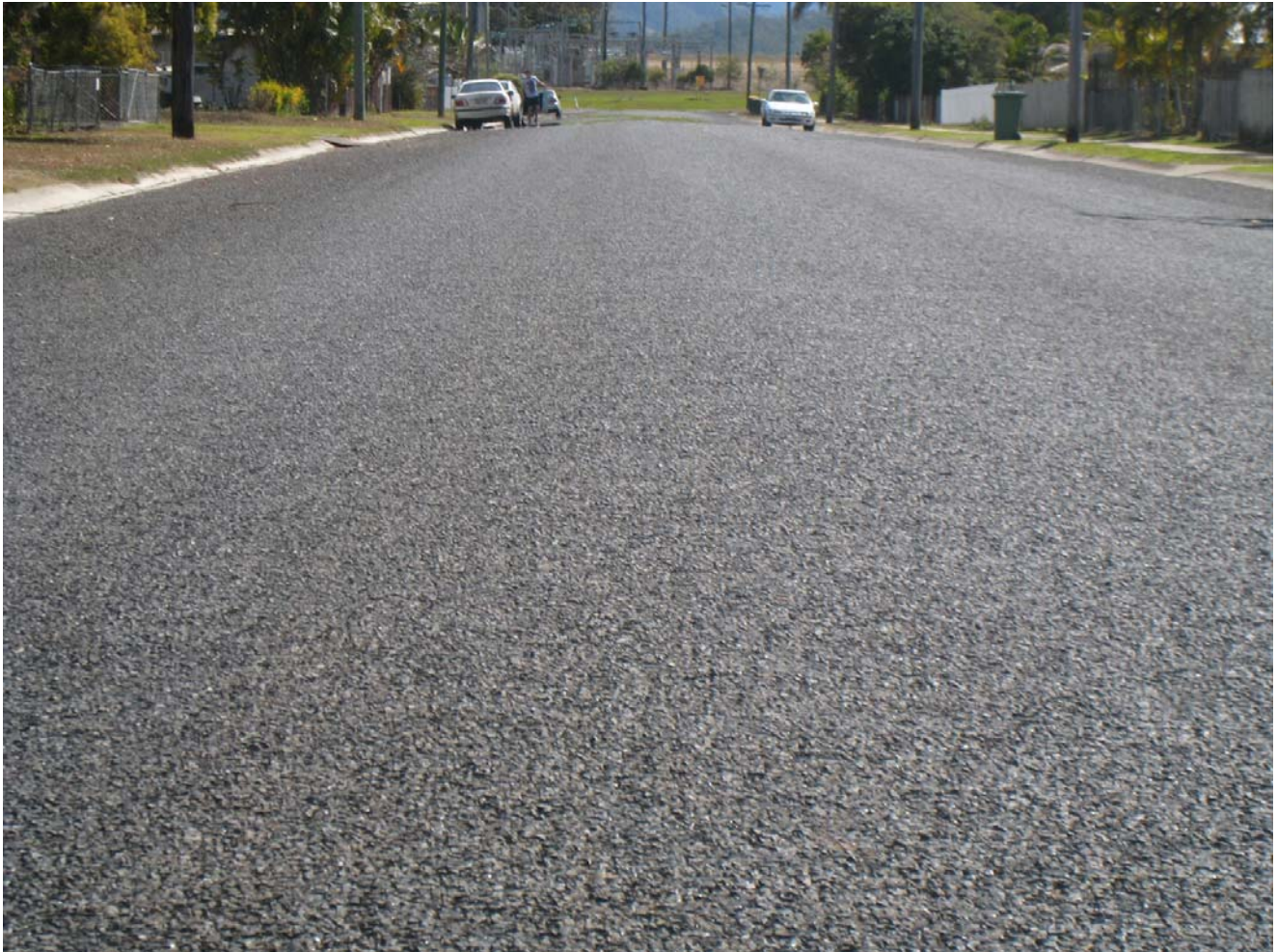
McIntyre Street Calen
