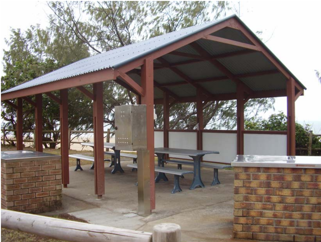
Sarina Beach Shelter Refurbishment – Southern Shelter
