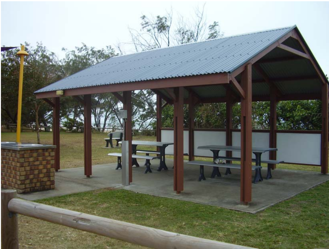
Sarina Beach Shelter Refurbishment – Northern Shelter
