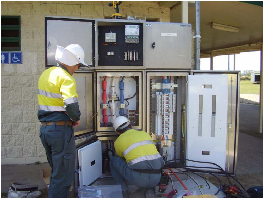
Norris Rd. Amenities/Sports Field Switchboard Replacement
