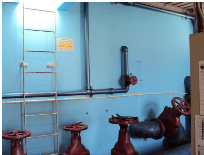
The repainted plant room
