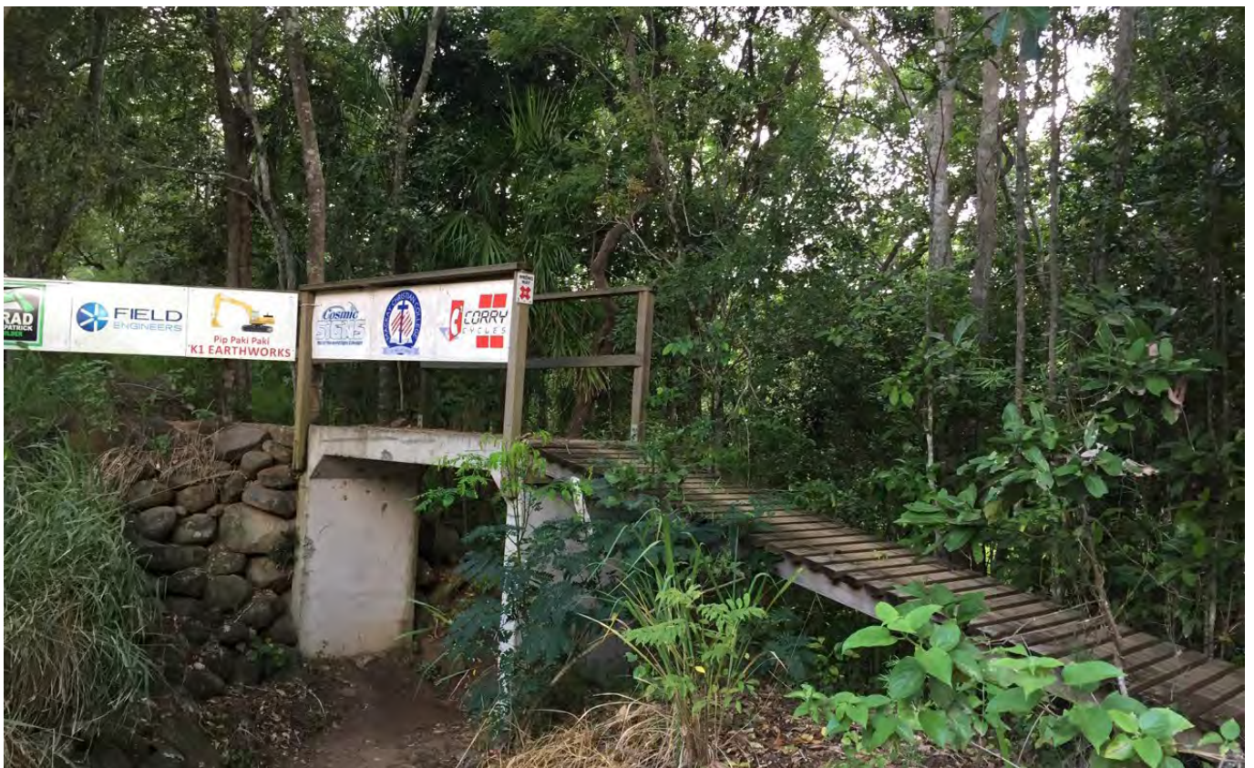
Figure 14. Bridge/crossover at Rowallan Park
