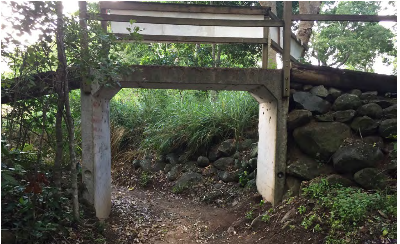
Figure 13. Bridge/crossover at Rowallan Park
