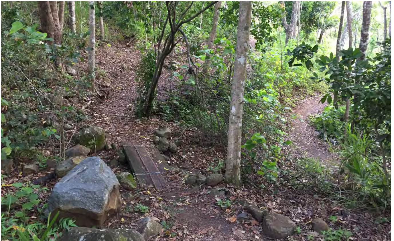
Figure 11. Typical bridge and rocky environment at Rowallan Park
